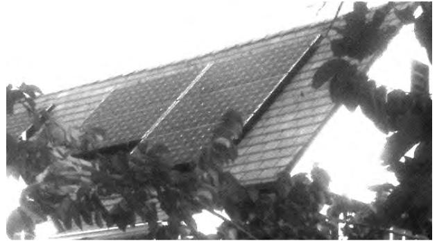
The photovoltaic panels themselves are fairly unobtrusive. As solar companies are usually focused on efficiency, sometimes the way the panels are racked and mounted can be problematic. Working with an architect can be one way to assure that your system is aesthetically pleasing, and the systems design also addresses waterproofing and structural issues.
