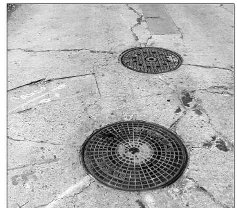
*An underground electricity vault in Oaks, probably installed in the 1930's. B.P. & L. stands for "Bureau of Power and Lighting." The ground has quite visibly shifted over the years.*
